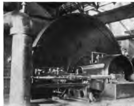
Fig. 2. Laminated Steel Fly-Wheel, 24' Diameter.*
